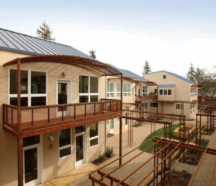
Florence Lofts in Sebastopol, California, features extensive energy-saving features.
